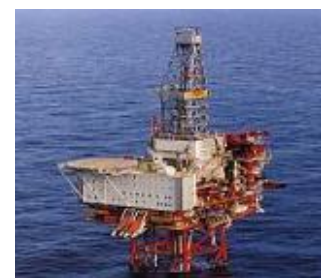
Well Head Platform
